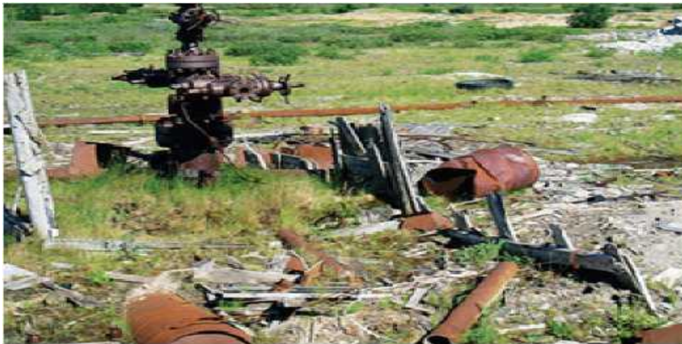
Figure 2 – Well considered abandoned
