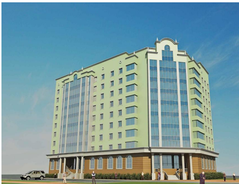
Figure 4 – Apartment building with 9 floors
